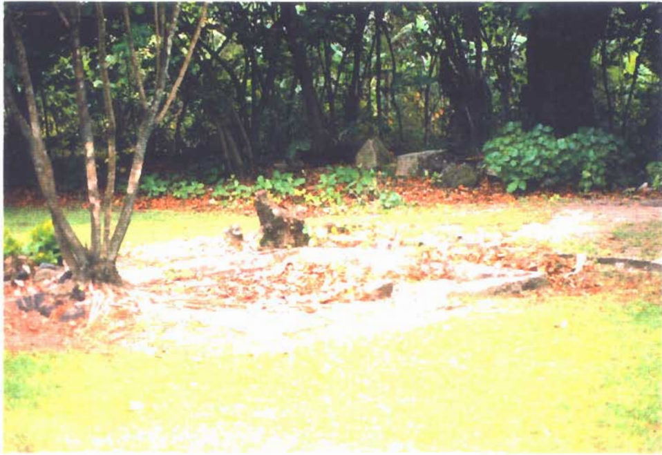
1. Concrete curbing, a floor slab, and footings located next to a parking lot and comfort station at the entrance to Kahana Valley State Park. View facing southwest.
