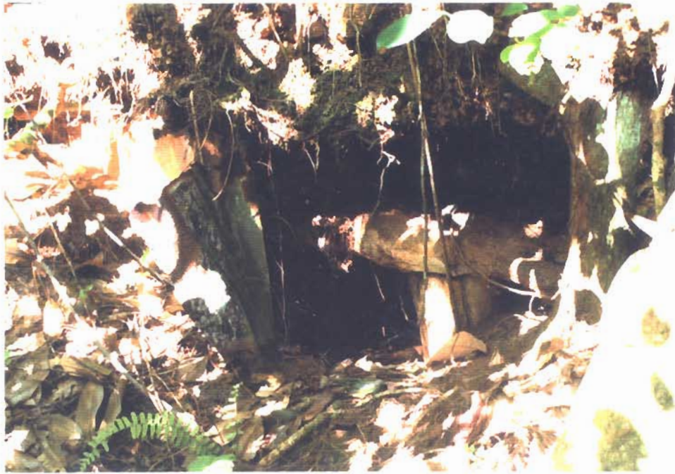
11. Corrugated sheet metal and timber bunker located along the side of Koolau Agriculture Company's irrigation system service road in Punaluu Valley.
