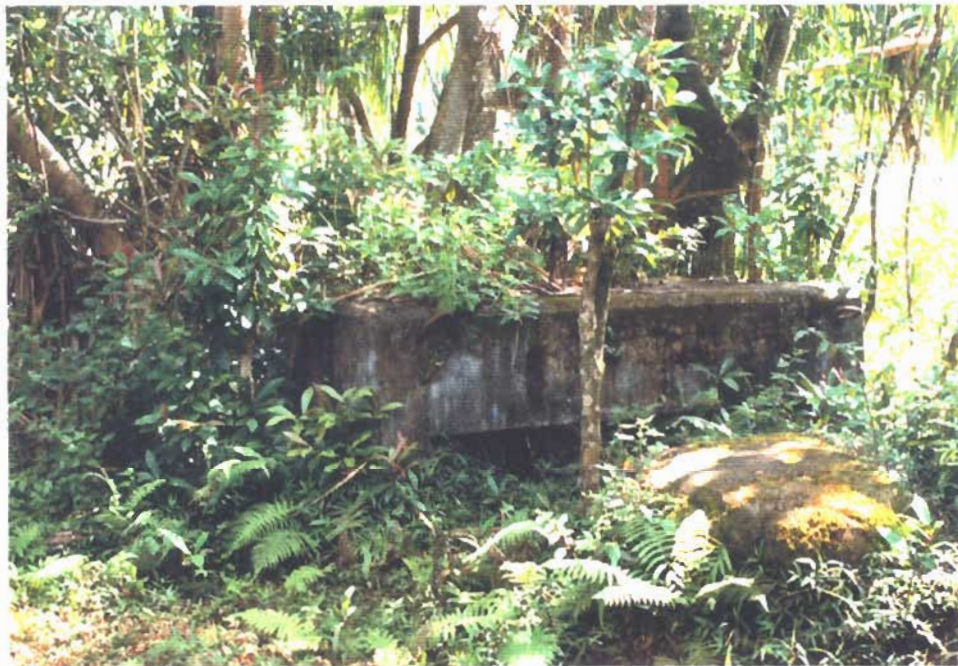
12. Quadrangular concrete bunker located near Koolau Agriculture Company's west irrigation ditch intake at Punaluu Stream.
