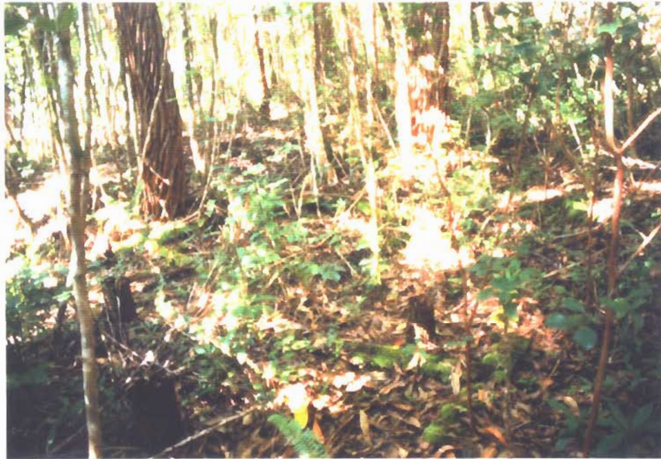
10. Upright timber footings to a military structure near the coral aggregate service road pictured above.
